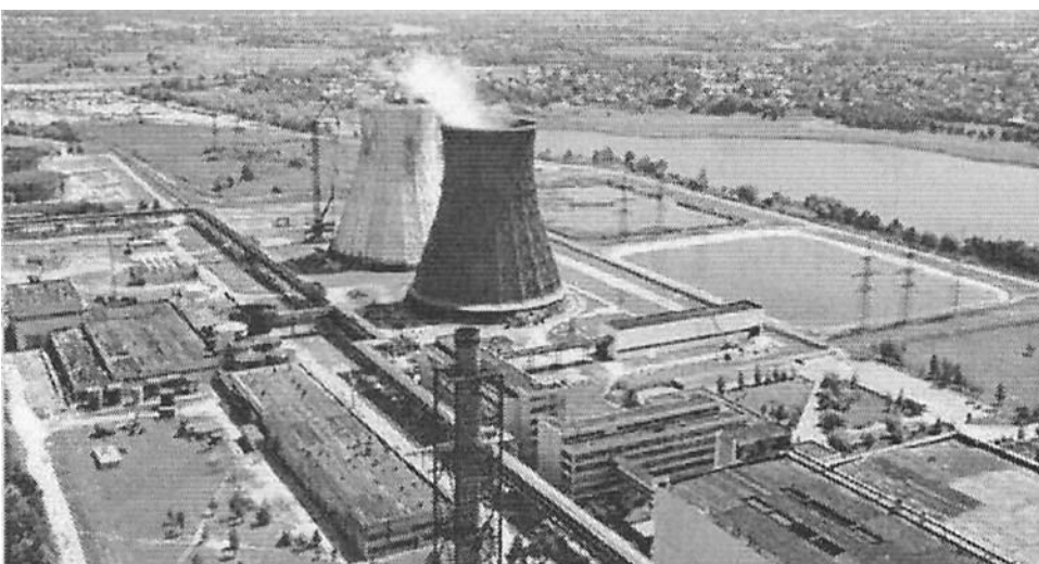
Fig. 3. The cooling system at the CHPP-5 (TEC-5) heating and power plant in Kharkiv, Ukraine. (Courtesy of Dr. Gennadiy K. Voronovsleyi, General Director.)
